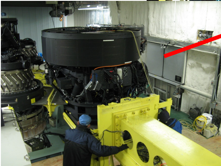
top unit exchange manipulating an 80t crane, Unit Loader, Man Basket, ...
